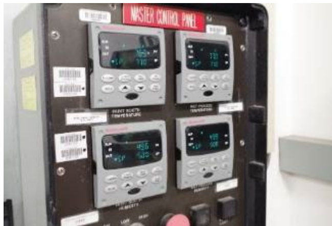
Figure 14: Controllers for Paint Mix Room and Spray Booth
